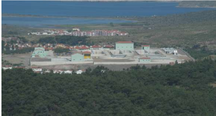
Küçükköy Municipality Wastewater Treatment Plant – Construction Year:2011 – Capacity: 111.426 m3/day
