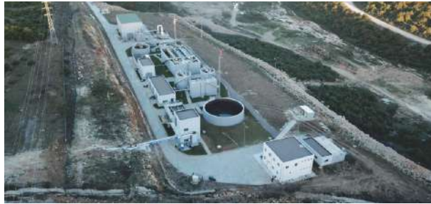
Makine İhtisas OIZ Municipal and Industrial WWTP – Construction Year:2016 – Capacity: 2.000 m3/day
