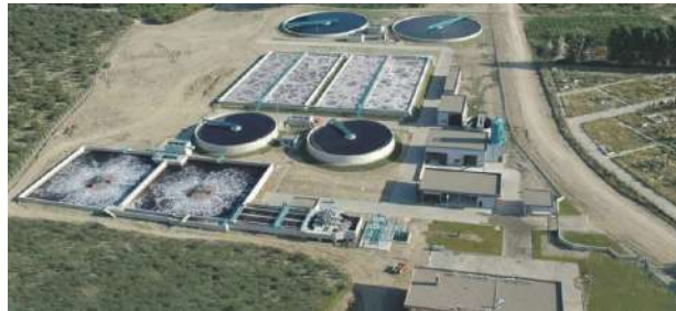
Yeşil Çevre OIZ Municipal and Industrial WWTP 1st Phase – Construction Year:2006 – Capacity: 52.500 m3/day
