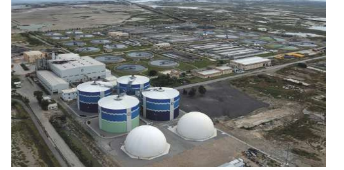
Çiğli Sludge Digestion ve Sludge Drying Plant –Construction Year:2014 – Capacity: 2.500 m3/day (Sludge Digestion)- 800 ton/day (Sludge Drying)
