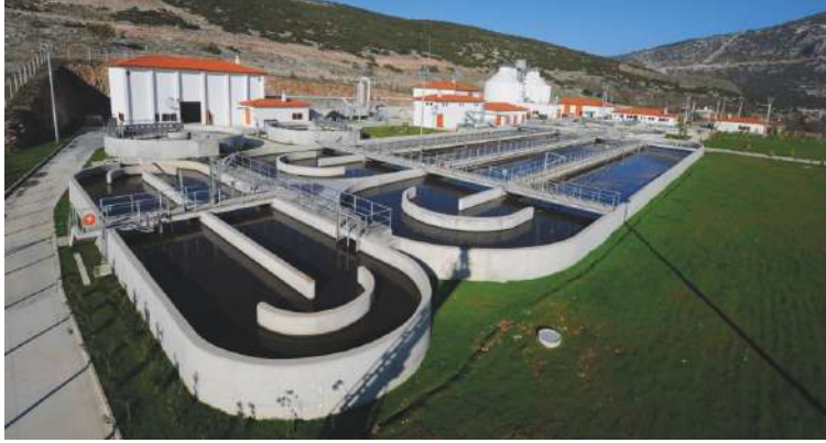
Muğla Wastewater Treatment Plant – Construction Year:2011 – Capacity: 17.111 m3/day
