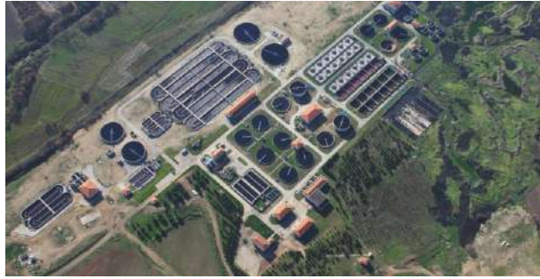
Çerkezköy OIZ Municipal and Industrial WWTP – Construction Year:2008 – Capacity: 80.000 m3/day
