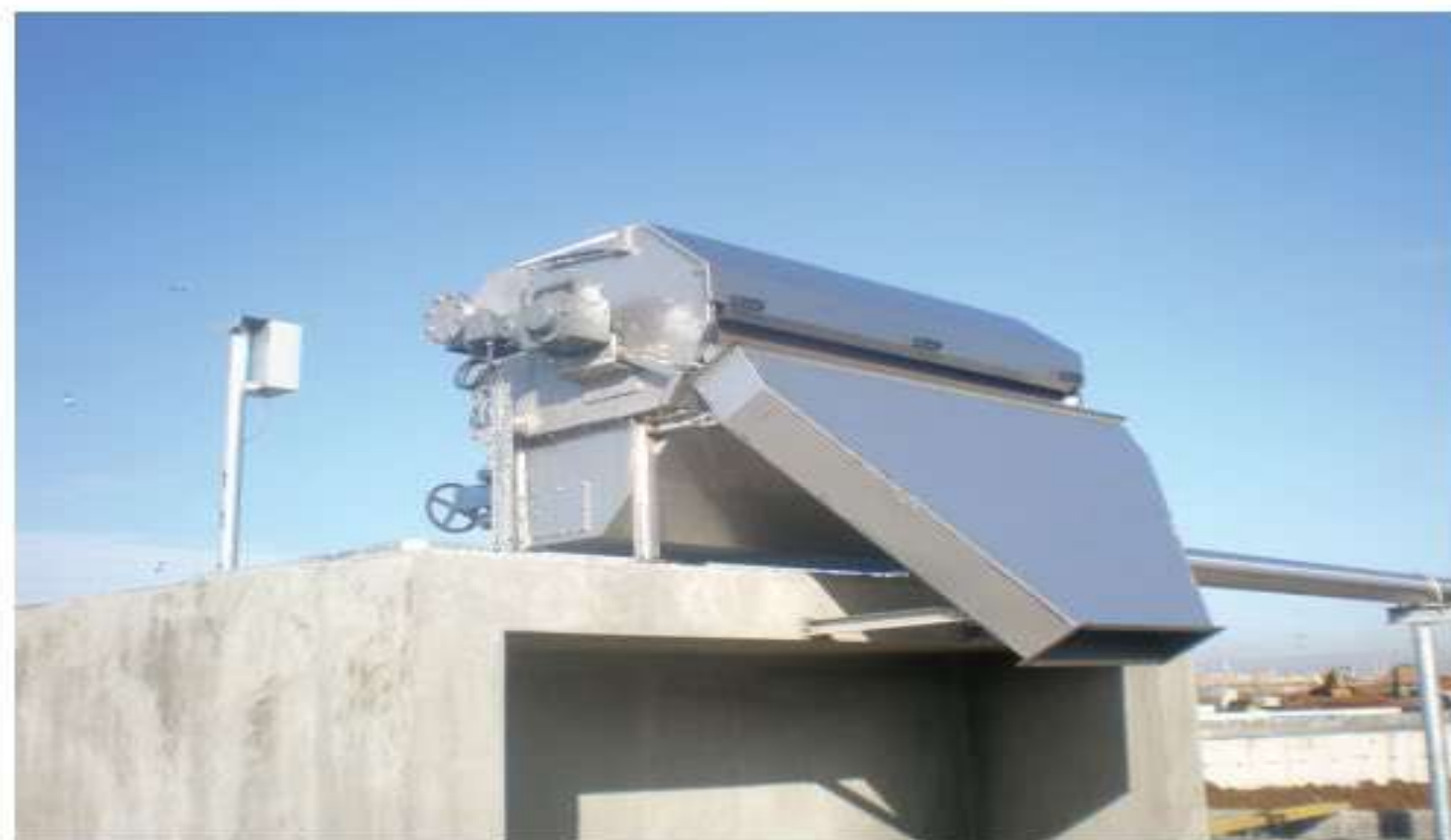
Completely enclosed Rotating Drum Screen
