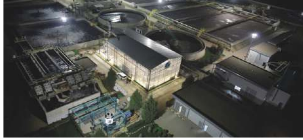
Yeşil Çevre OIZ Municipal and Industrial WWTP 2nd Phase- Construction Year:2015 – Capacity: 150.000 m3/day
